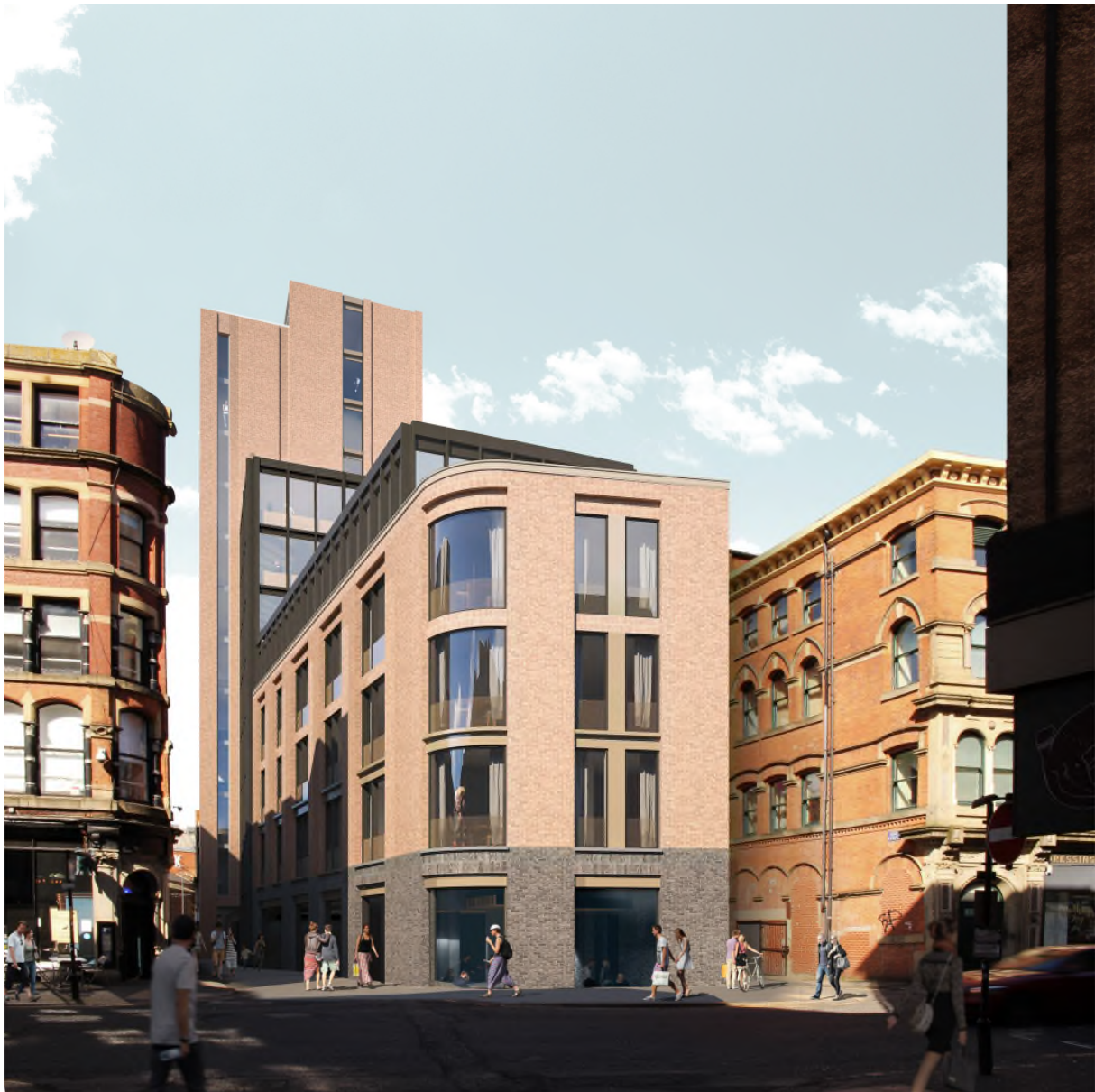
Viewpoint 3: from the junction of Back Turner Street and High Street, looking north towards the application site
